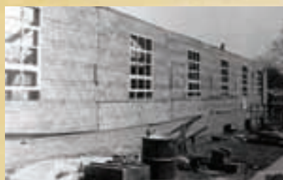
Getting started on new sanctuary Summer 1964
