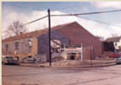
Church Auditorium under way 1964
